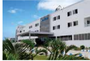
Rudrapur Plant (Green Building)
