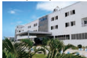
Rudrapur Plant (Green Building)
