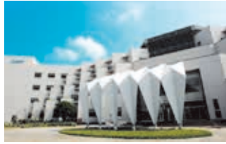
Tainan Plant (Diamond-rated Green Building)
