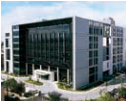
Taoyuan Technology Center (Green Building)
