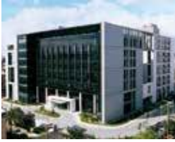
Taoyuan Technology Center (Green Building)
