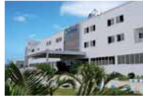
Rudrapur Plant (Green Building)
