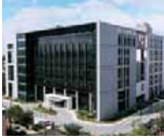
Industrial Center renewable energy
